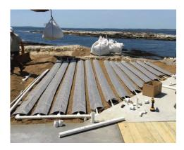
► GeoMat<sup>™</sup> is the lowest profile system for sites limited by ledge, water table or impermeable soils.
