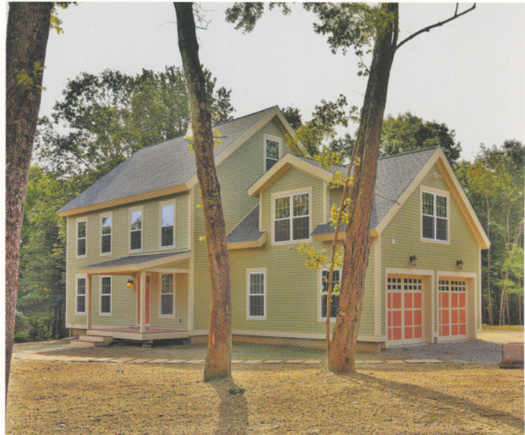
Ark Contractors HERS 35
