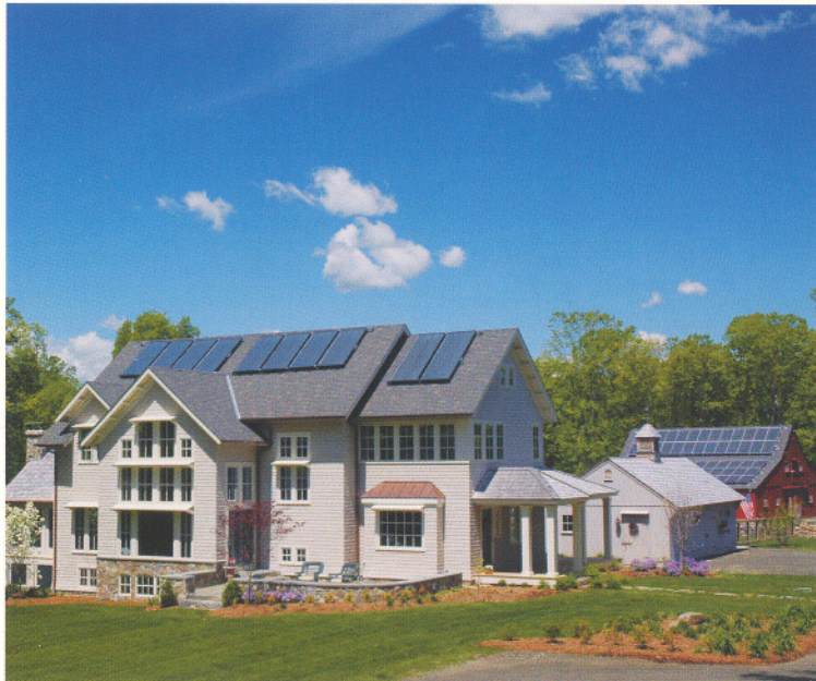
Consulting Engineering Services HERS-7
