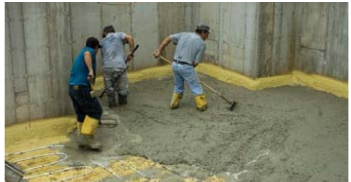
Concrete is being spread over radiant coils.
