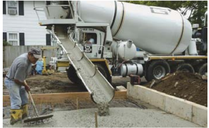
Pouring the basement floor O&G concrete with recycled glass for added strength. Wire mesh and spray foam over the trap rock for insulation.
