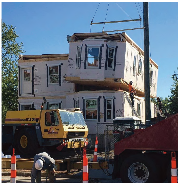
Westchester modular units being installed
