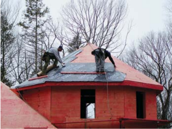
Bridgewater shop building ice & water shield.
