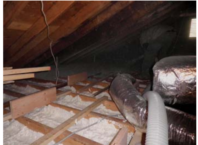
Adding cellulose over foam in attic floor to meet prescribed R-value.
