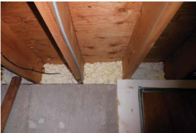
Foamed rim joist in basement.
