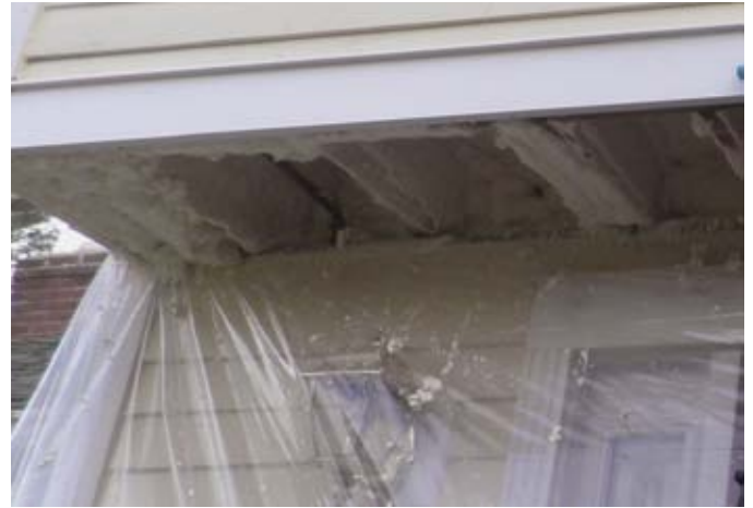
Foam sprayed in cantilevered floor accessed by removing soffit.
