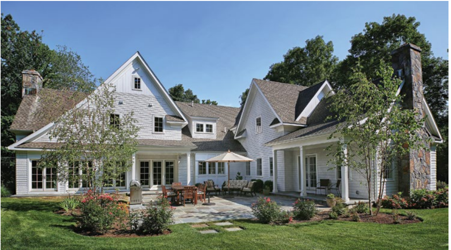
DeRoas Builders Darien custom home
