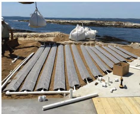
► GeoMat™ is the lowest profile system for sites limited by ledge, water table or impermeable soils.
