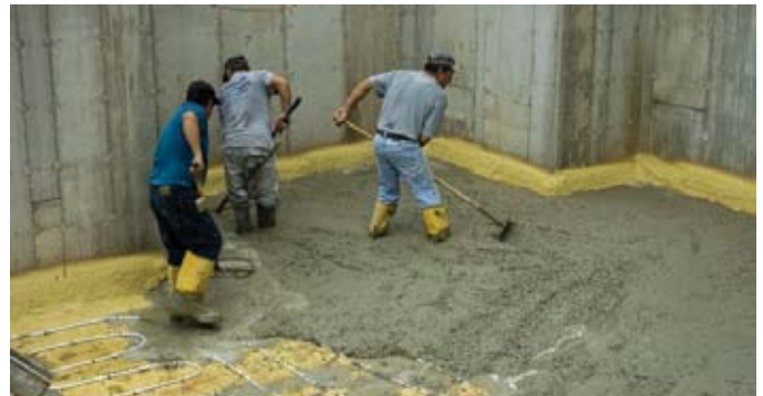
Concrete is being spread over radiant coils.
