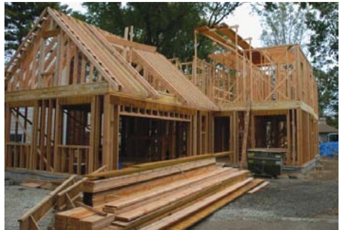
Performance House being framed.
